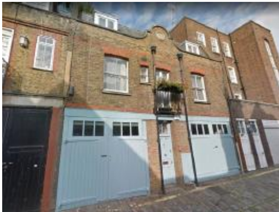
Photograph 4: Front elevation of 19 Wigmore Place
