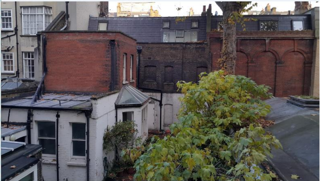
Photograph 3: View towards the rear of 19 Wigmore Place
